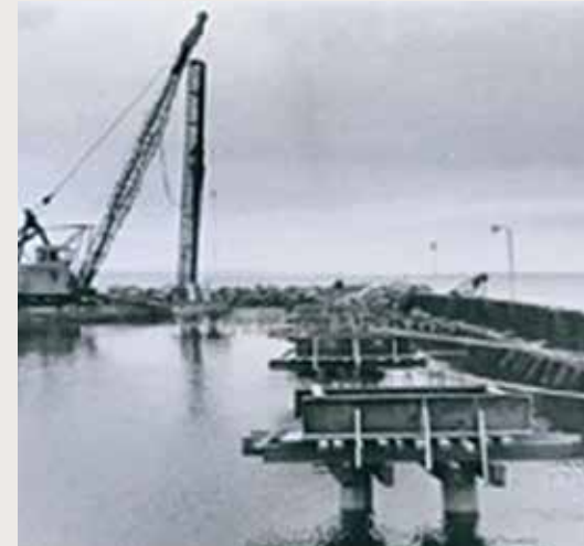
1976 building of the Edmonds Fishing Pier
